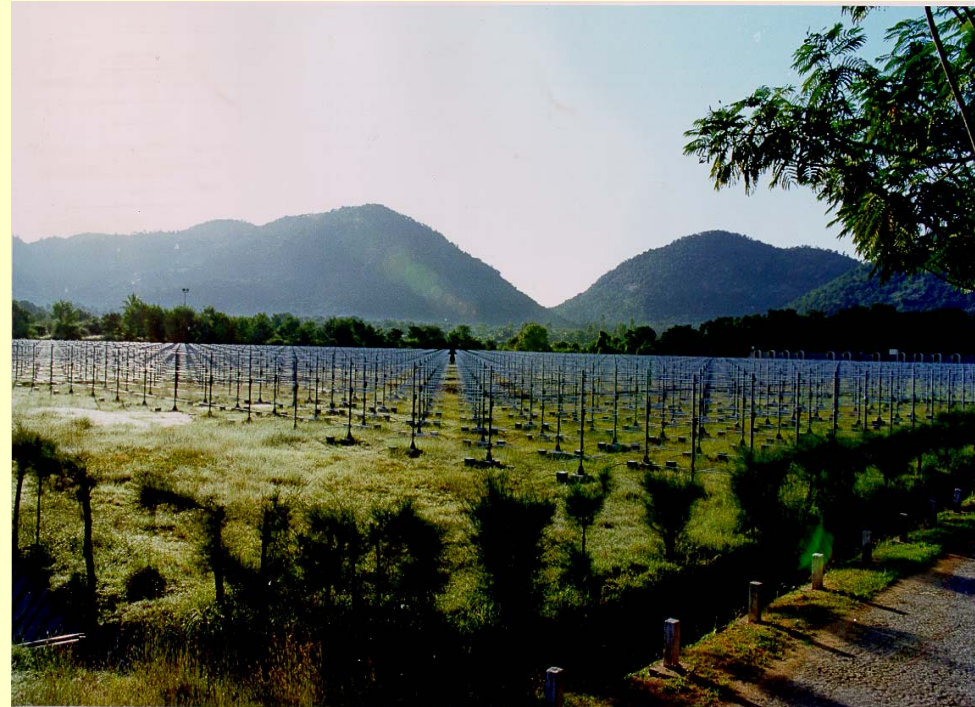
32X32 Yagi Antenna Array of MST Radar
